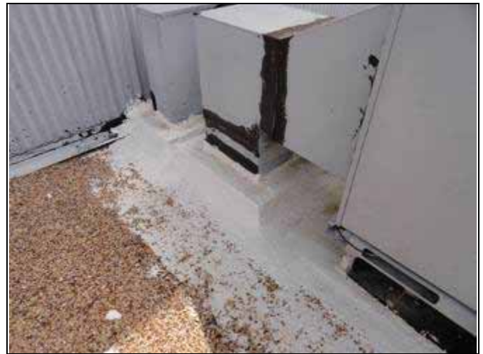
22. Equipment flashing at built-up roof
