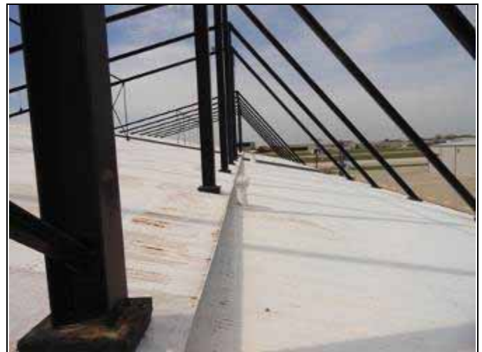
12. North roof at 4730
