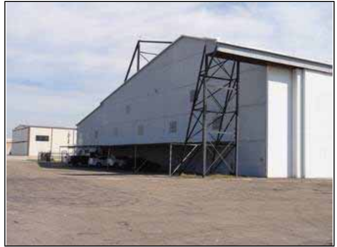
2. Left side, west elevation of 4726
