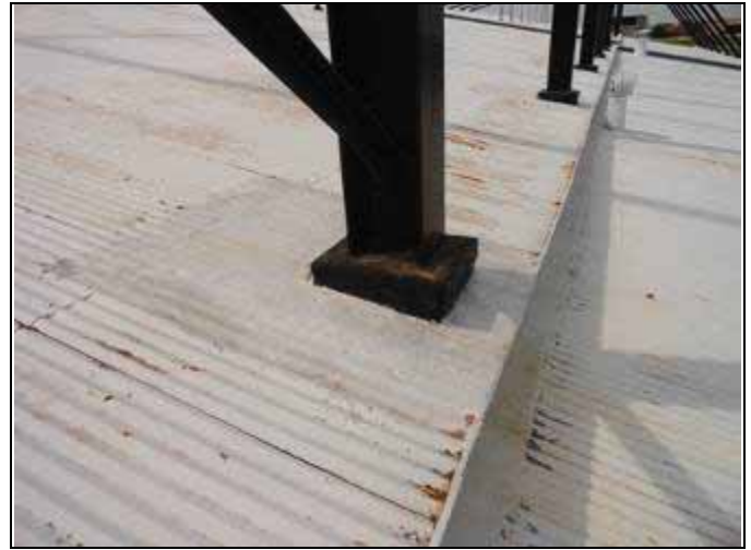
68. Repaired flashing at structural penetration
