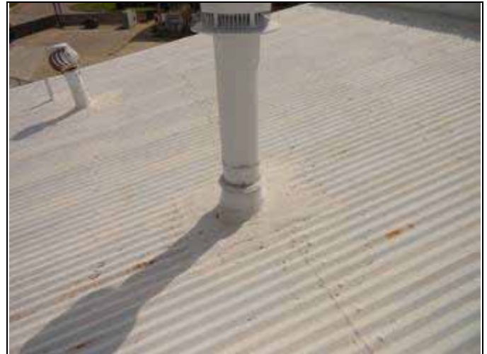
18. Plumbing penetration at roofs
