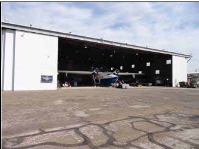
5. Front, south elevation of 4730
