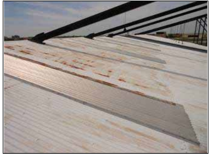
20. Skylight replacement panel at 4730
