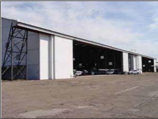
1. Front, south elevation of 4726
