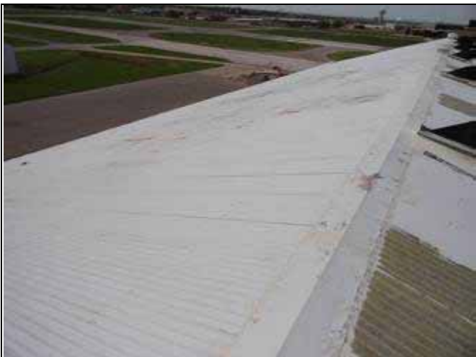
11. South roof at 4726
