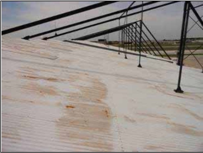
13. North roof at 4730
