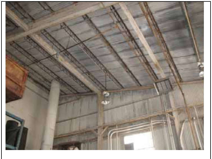
4. View of roofing underside in east hanger.
