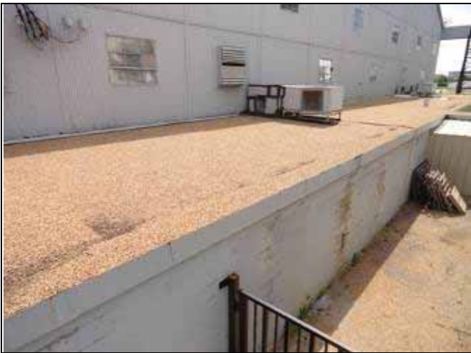
21. Built-up roof west of 4730
