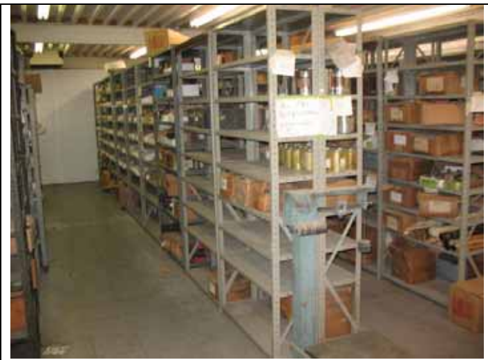
5. View of west side storage area with ACBM floor tile/mastic.
