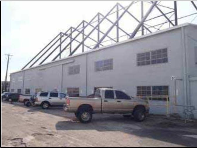
7. Rear, north elevation of 4730
