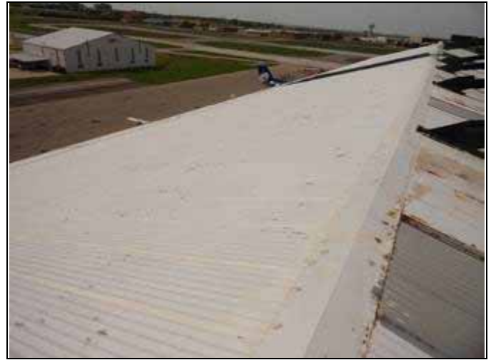
14. South roof at 4730
