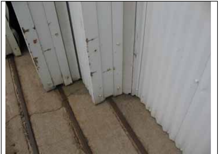
24. View of door gaskets on south hanger doors of west hanger.
