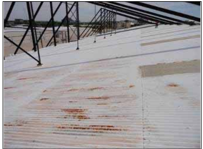
10. North roof at 4726
