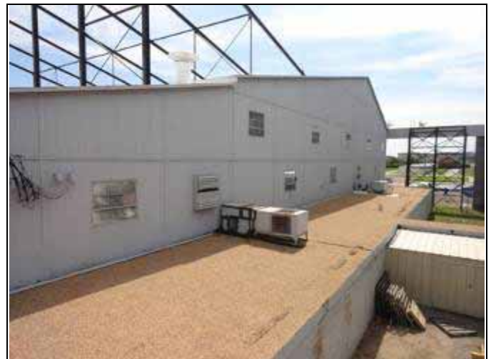
6. Left side, west elevation of 4730
