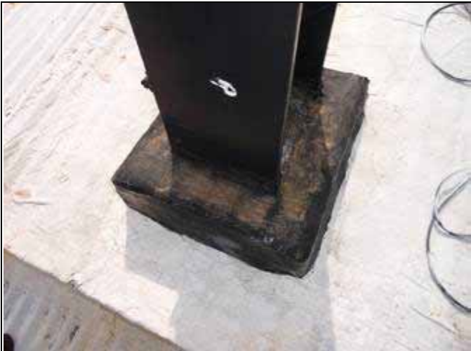
17. Structure penetration at roofs
