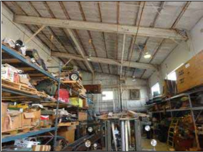
49. Rear hangar interior
