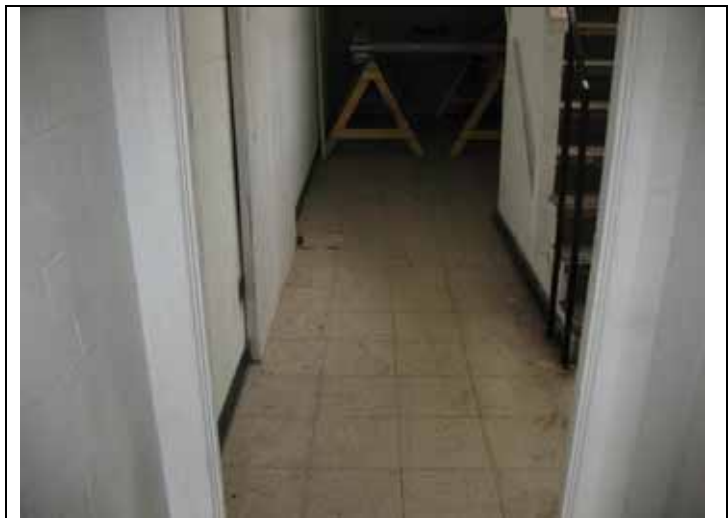
18. View of connecting hallway.
