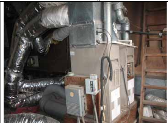
11. View of 2 nd floor mechanical room in east hanger.
