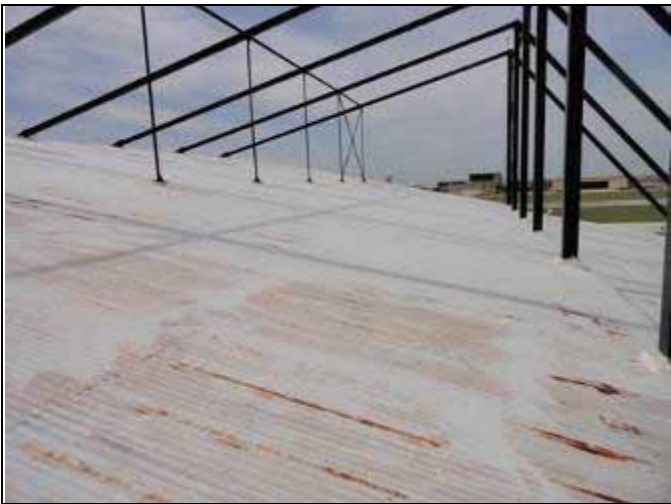
9. North roof at 4726
