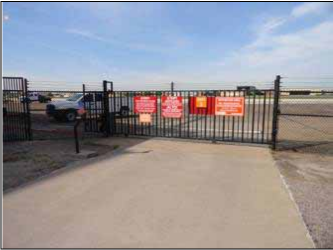
25. Secured airport access gate
