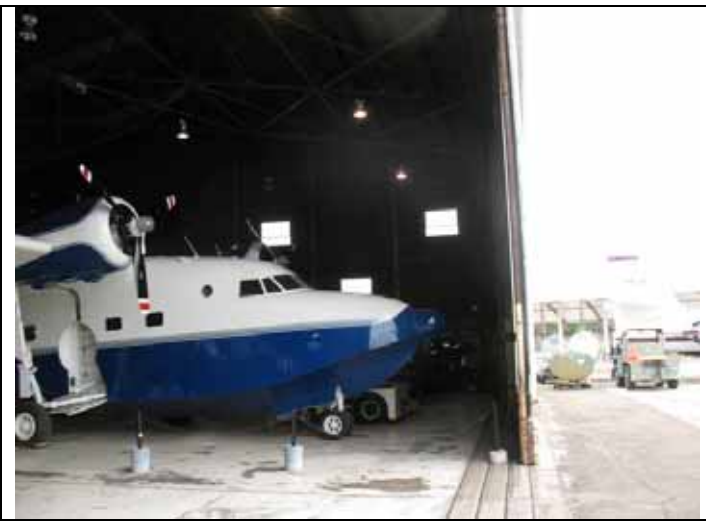
1. View to the east across south hanger doors of East Hanger.
