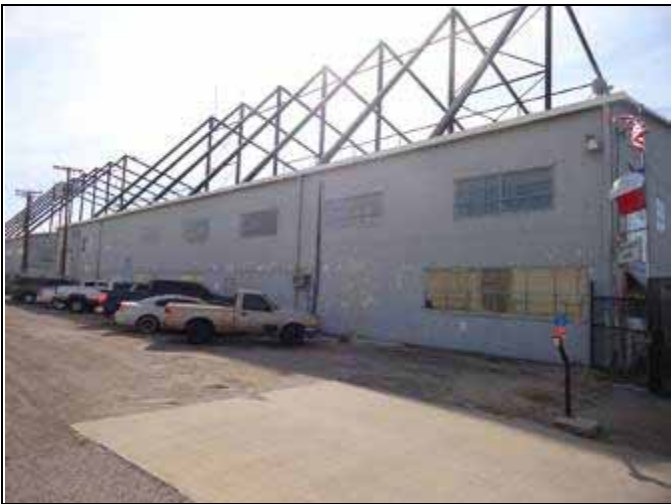
3. Rear, north elevation of 4726
