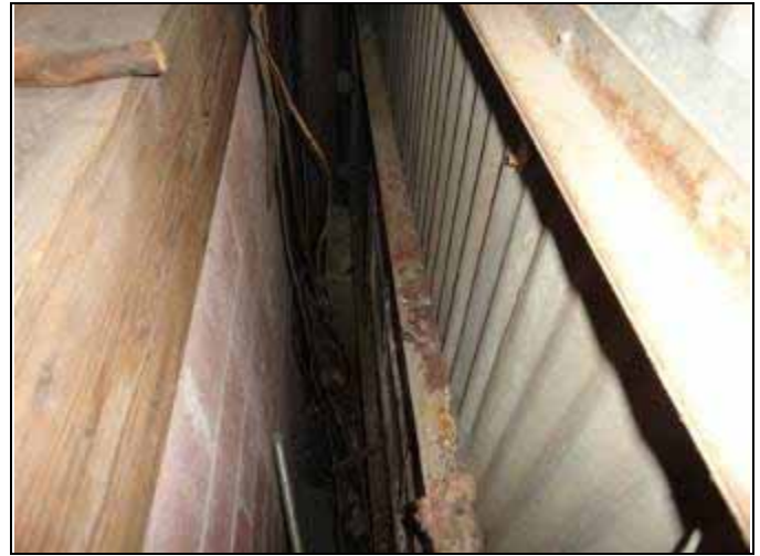
32. Interstitial space between occupied areas and exterior walls
