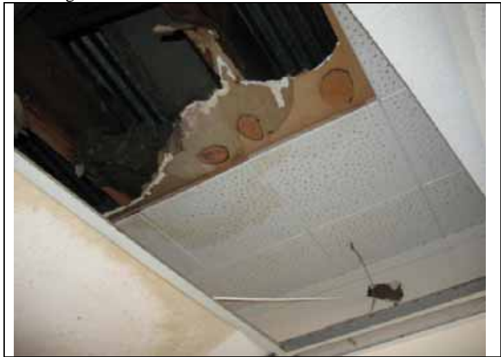
10. View of ACBM ceiling mastic in 2 nd floor room above NE office area in east hanger.
