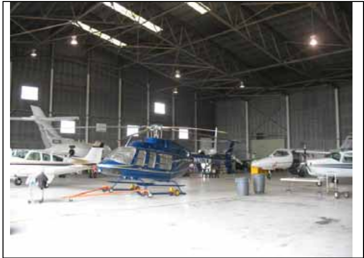
14. View of north interior of west hanger.
