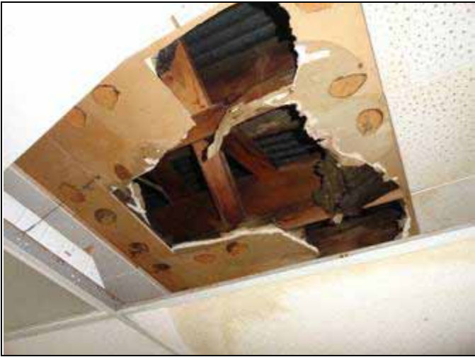
31. Upper ceiling framing at mezzanine areas
