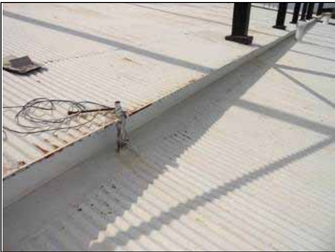
15. Step transition at roofs
