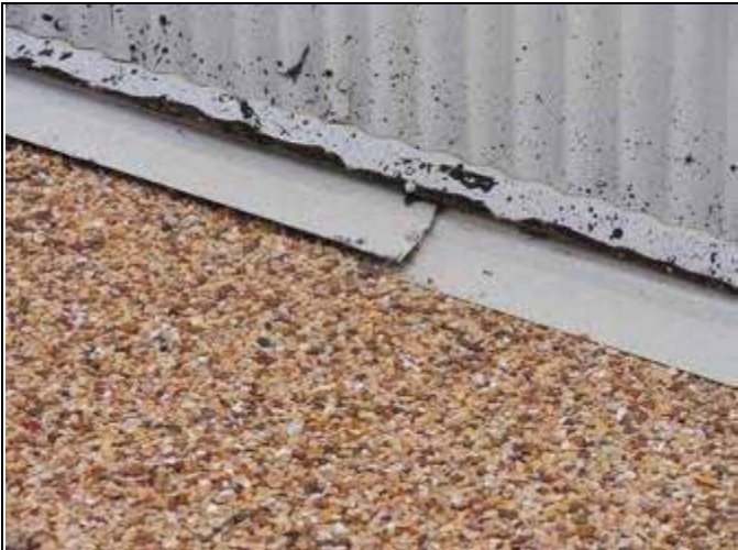
23. Flashing at roof transition to wall panel
