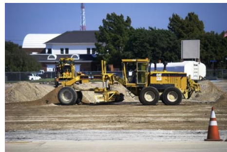
Above: new dirt being spread at the Sky B&B site.
