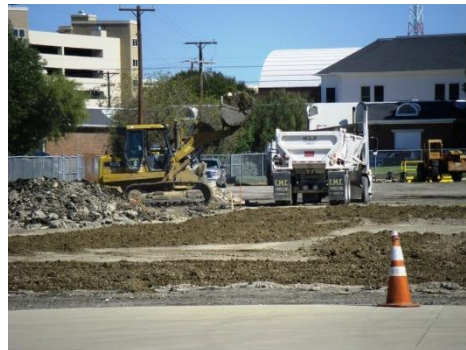
Below: old dirt and pavement being hauled away.
