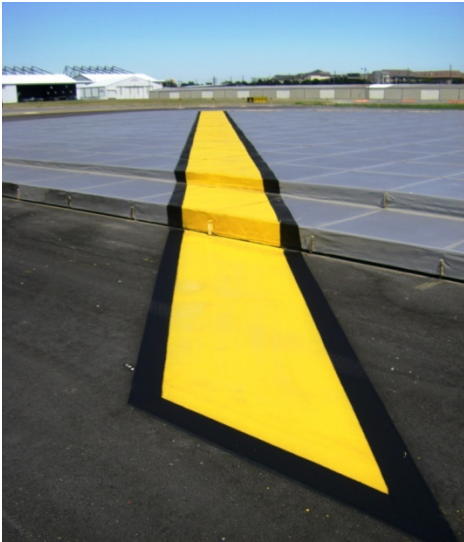
Above: a view of the completed EMAS.
