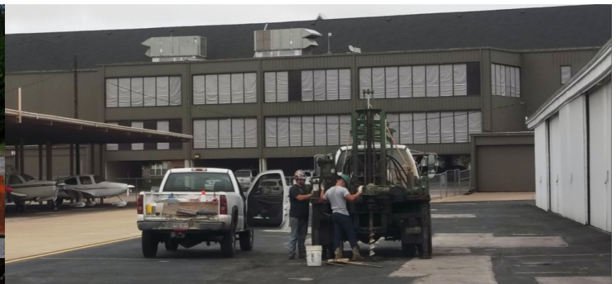
Above Left: asphalt that was badly rutted by the garbage trucks servicing this dumpster at 4700 Airport Parkway was replaced with 10-inch thick concrete. Left: failed asphalt in the driveway at 4700 Airport Parkway was also removed and replaced. Above: a geotechnical crew takes core samples from the ramp at the S4 T-hangars. The ramp is in extremely poor condition and will be reconstructed this fiscal year. Right: a Town of Addison crew “pot-boling” the water line that runs underneath Taxilane Victor, in preparation for the reconstruction project scheduled to start in spring 2015.
