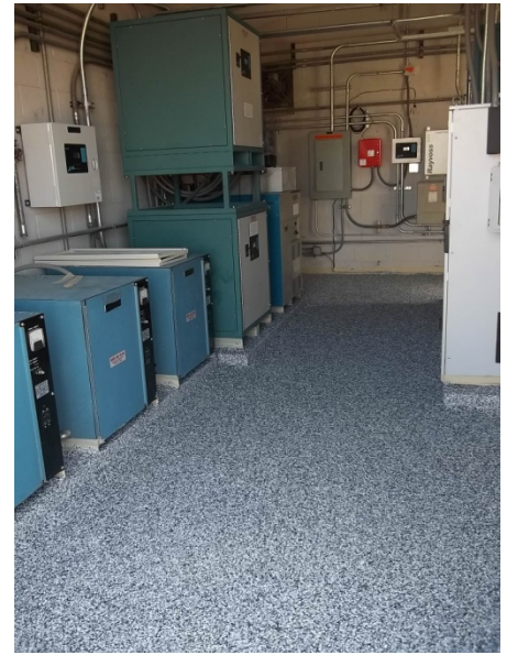
Above: the floor of the airfield lighting and control vault was unfinished concrete (left); the center photo shows the floor being prepared for an epoxy finish, and the photo at right shows the finished product. The floor coating will aid Airport Maintenance in keeping the vault clean and relatively dust-free, which in turn is beneficial for the electrical equipment – the airfield lighting regulators and control circuits – housed in the vault.
