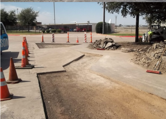
Above Left: asphalt that was badly rutted by the garbage trucks servicing this dumpster at 4700 Airport Parkway was replaced with 10-inch thick concrete. Left: failed asphalt in the driveway at 4700 Airport Parkway was also removed and replaced. Above: a geotechnical crew takes core samples from the ramp at the S4 T-hangars. The ramp is in extremely poor condition and will be reconstructed this fiscal year. Right: a Town of Addison crew “pot-boling” the water line that runs underneath Taxilane Victor, in preparation for the reconstruction project scheduled to start in spring 2015.
