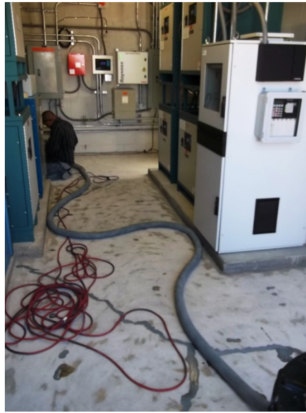
Above: the floor of the airfield lighting and control vault was unfinished concrete (left); the center photo shows the floor being prepared for an epoxy finish, and the photo at right shows the finished product. The floor coating will aid Airport Maintenance in keeping the vault clean and relatively dust-free, which in turn is beneficial for the electrical equipment – the airfield lighting regulators and control circuits – housed in the vault.
