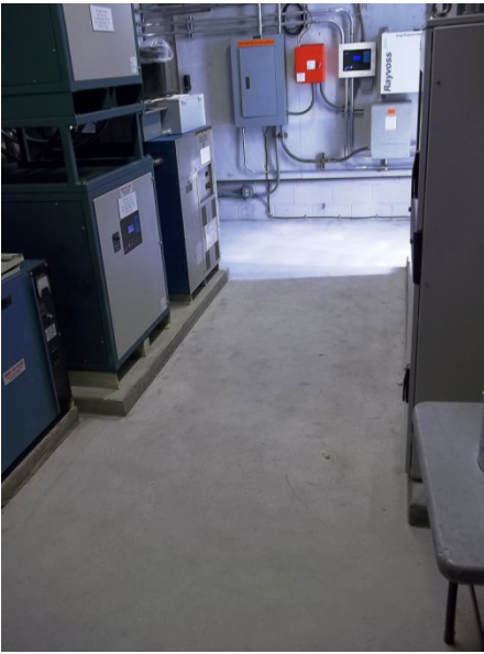
Above: the floor of the airfield lighting and control vault was unfinished concrete (left); the center photo shows the floor being prepared for an epoxy finish, and the photo at right shows the finished product. The floor coating will aid Airport Maintenance in keeping the vault clean and relatively dust-free, which in turn is beneficial for the electrical equipment – the airfield lighting regulators and control circuits – housed in the vault.
