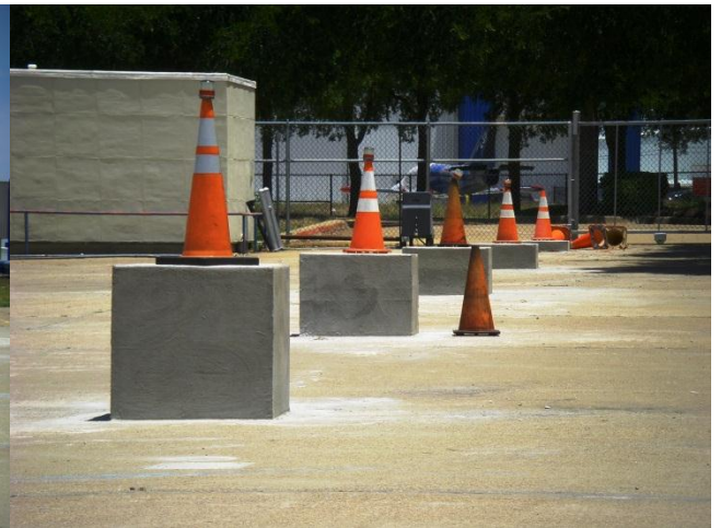
Concrete pilings and piers have been set in place on the north side of the Jetport ramp (fronting Taxiway Alpha, immediately south of Taxiway Victor). These piers will support a steel-frame canopy structure which will provide interim shelter for a Boeing Business Jet (BBJ) pending completion of a permanent hangar complex just south of Taxiway Sierra. Steel for the interim structure will arrive in mid-July, after which construction is expected to move very quickly.
