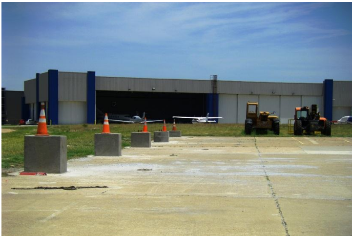
Concrete pilings and piers have been set in place on the north side of the Jetport ramp (fronting Taxiway Alpha, immediately south of Taxiway Victor). These piers will support a steel-frame canopy structure which will provide interim shelter for a Boeing Business Jet (BBJ) pending completion of a permanent hangar complex just south of Taxiway Sierra. Steel for the interim structure will arrive in mid-July, after which construction is expected to move very quickly.
