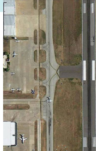
Taxiway Hotel intersection, August 2, 2012
