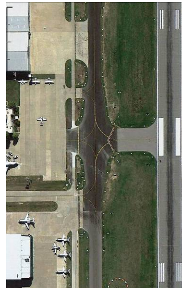
Taxiway Hotel intersection, October 18, 2013
