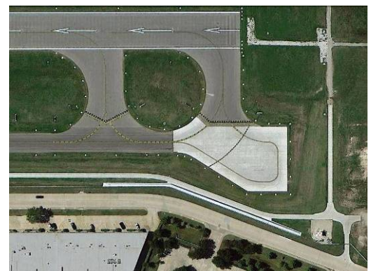
North end of Taxiway Alpha, October 18, 2013
