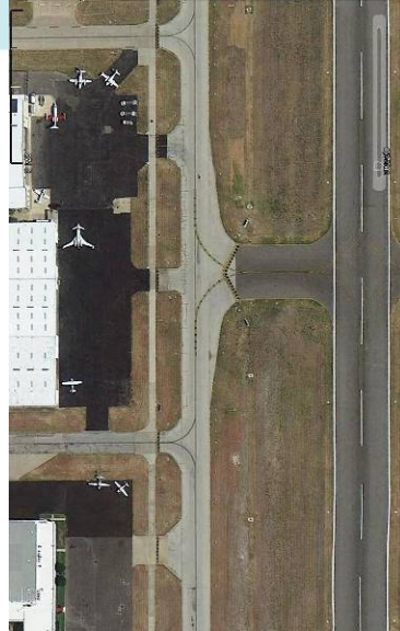
Taxiway Foxtrot intersection, August 2, 2012
