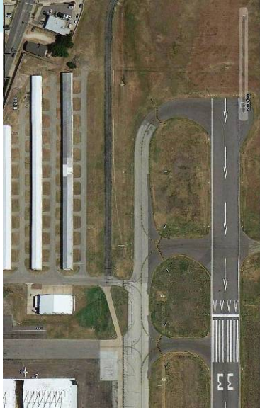
South end of Taxiway Alpha, August 2, 2012
