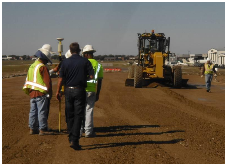
Recent construction activity on Taxiway Alpha ... Above: workers forming concrete for a drainage inlet structure. Right: grading and surveying the base for Stage VII. Below: rolling in the base on Stage VII.
