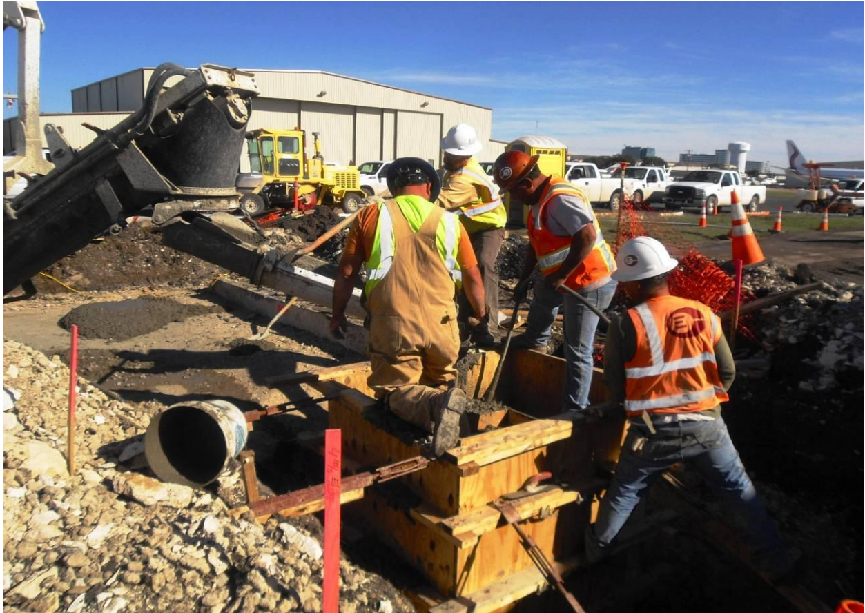
Recent construction activity on Taxiway Alpha ... Above: workers forming concrete for a drainage inlet structure. Right: grading and surveying the base for Stage VII. Below: rolling in the base on Stage VII.
