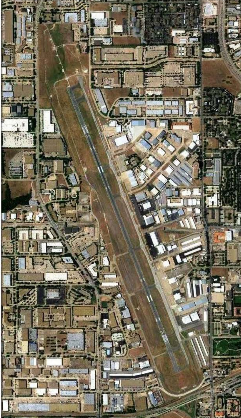
Figure A-3: Aerial photo of airport (August 2, 2012 image from Google Earth).
